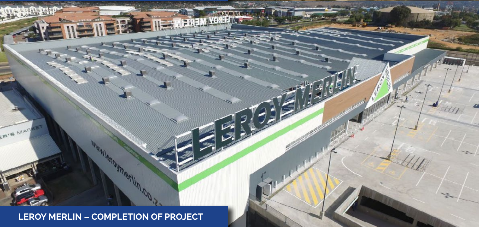
MASSBUILD RDC - COMPLETION OF PROJECT
